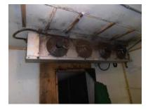
Immediate Action Required - There is a rear cooler room that is in poor condition. The ceiling has fallen as a result of moisture from within. Have a contractor determine needed repairs and costs.
