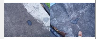
**Attention Needed** - The detached garage roof covering material needs some repair to prevent further deterioration or water leakage.
