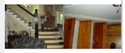
Satisfactory - The main staircase is appropriately installed. The staircase has a landing. There was separation noted between the staircase and wall at the landing level.
