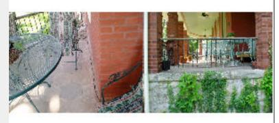
**Action Necessary** - The entry porch needs repair or replacement due to deterioration or settlement. The settling porch has moved to the point that major repair, or mud jacking is needed to prevent water from collecting and settling the soil under the porch further. Estimates from qualified professionals are called for.
