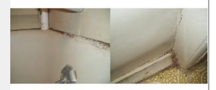
**Attention Needed** - The caulking in the water contact areas appears to need attention. Damage may result if not corrected. The seam where the tub or the shower meets the flooring needs to be caulked to prevent damage. The wall - tub or shower seam needs to be caulked to prevent moisture from entering the wallboard.
